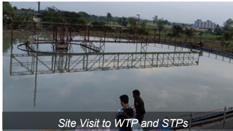
Site Visit to WTP and STPs
